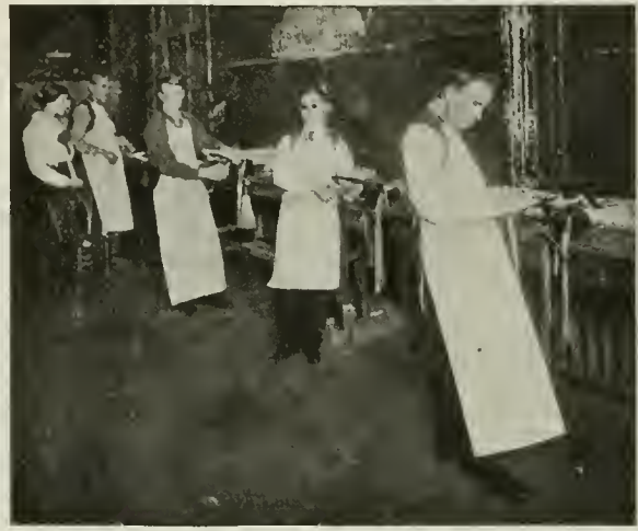
Some Idea of the Work Done by the Blind May Be Judged from This View, Where All Sorts of Intricate Coils Are Wound and Taped.
